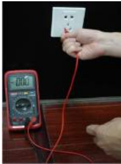
Appendix Figure 7-7 Check neutral cable connection
