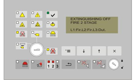
Turn the switch to position *Manual* to enable the extinguishing and the evacuation time to be counted down again.
