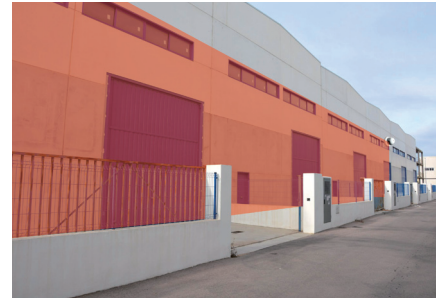
Wall protection (outdoor) at Warehouse
